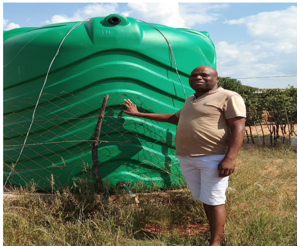
Bushy Mamba, a community member from Lusaka Village in Moutse, standing next to the empty water storage tank that was installed in November 2020. Sekhukhune District Municipality haven't provide water in the tank since its installation
